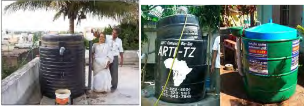
Figure 7 – Household floating drum digesters
