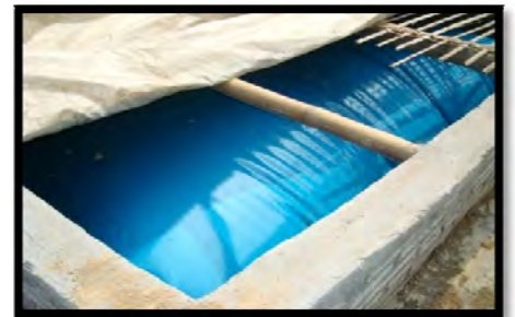
Figure 21 – Chongqing Xinshui 15m 3 Digester
