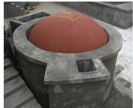
Figure 20 – ACME 10m 3 Digester
