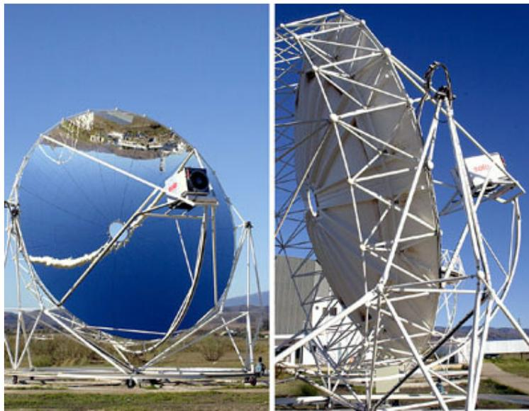
**Figure 5.2: Solar dish/Stirling engine system (from PSA website)**
